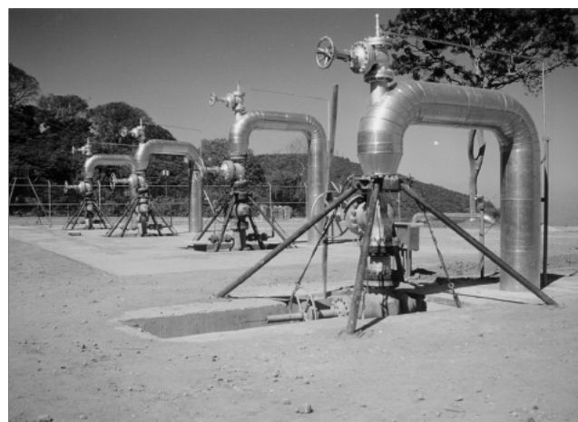
Fig.3 TR-5 wellhead
