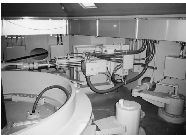
Fig.6 Electric deflector servomotor
