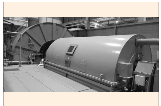
Fig.2 Steam turbine and generator for the 75-MW biomass power plant
