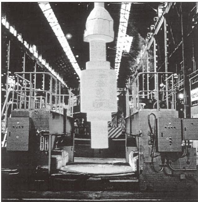
Fig.3 Intermediate-pressure internal casing under construction
