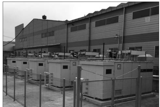
Fig.8 Delivered phosphoric acid fuel cells
