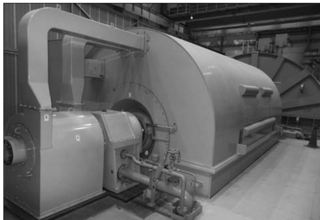
Fig.3 Steam turbine and generator for 2nd Nagoya Power Plant
