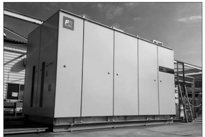
Fig.7 Solid oxide fuel cell for commercial use (prototype system)
