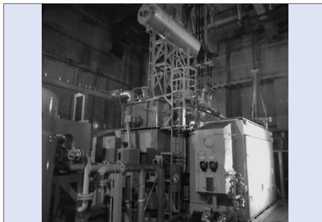
Fig.5 Transformer rectifier for DC furnaces
