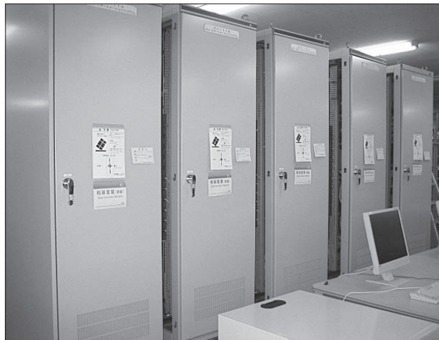
Fig.1 MICREX-NX panels for an independent power producer
