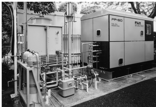
Fig.7 Fuel cell for biogas
