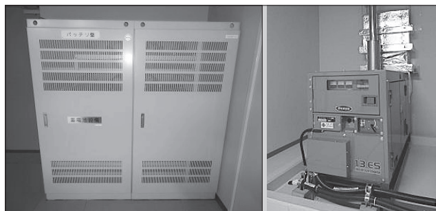
Fig.2 Installed state of backup power supply equipment
