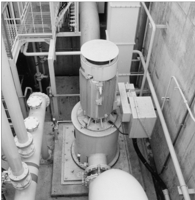
Fig.10 Exterior view of the hot well pump
