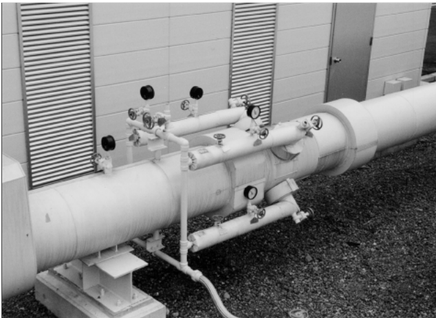
Fig.5 Exterior view of the venturi tube
