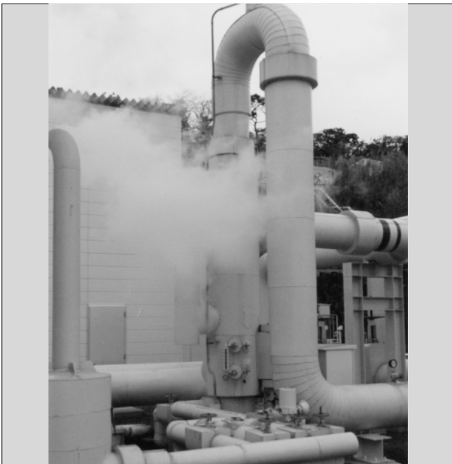
Fig.6 Exterior view of the mist separator
