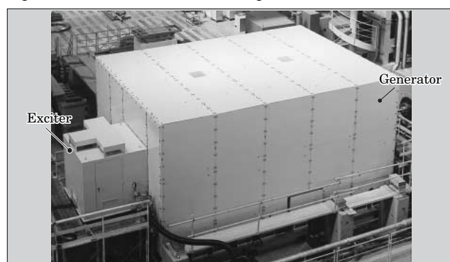
Fig.1 280 MVA air-cooled turbine generator
